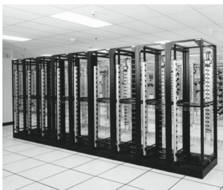
Equipment frames with CableControl installed
